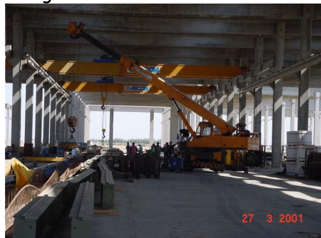
Bridge Crane Installation
