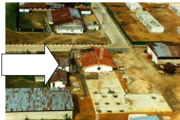
Aba road, box offices under construction
