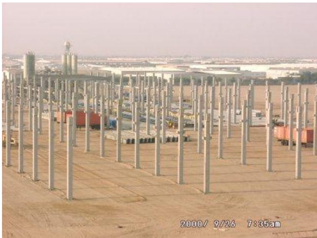
Aerial View PRECO Factory
