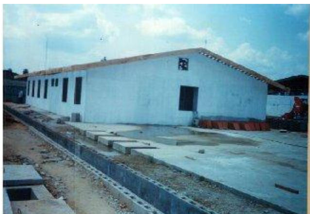
850 sqm pre-cast offices built in 60 days, 01/feb/98 - 01/apr/1998
