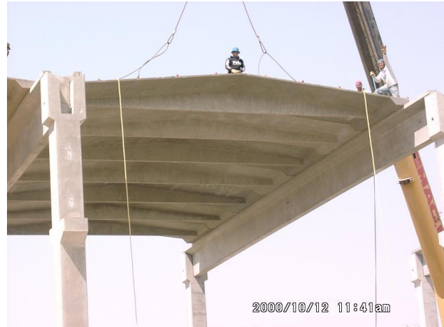
Seagull Roof Erection
