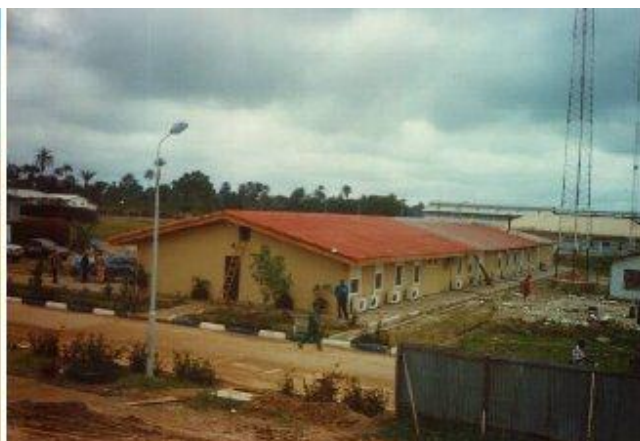
850 sqm pre-cast offices built in 60 days, 01/feb/98 - 01/apr/1998
